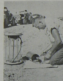
Paul Schabacker checks compacted fill for density determination using water-ballooning method at the new City of Phoenix reservoir; a typical step in testing and control by Engineers Testing Laboratories, Inc.
