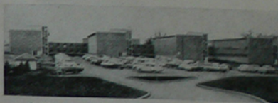
12,200 square feet of Porcelo Panels were used in the construction of the New Engineering Buildings at Colorado A. & M. College.
